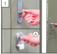
**TO CLOSE** ;- With the doors in the open position, fix together holding the doors together and turn the cylinder thumb turn (inside) or the key (outside) on door 'A'. This will engage both doors together and can now be closed as one door on the top latch.
