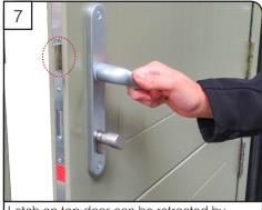
Latch on top door can be retracted by handle or cylinder to release the combined door.
